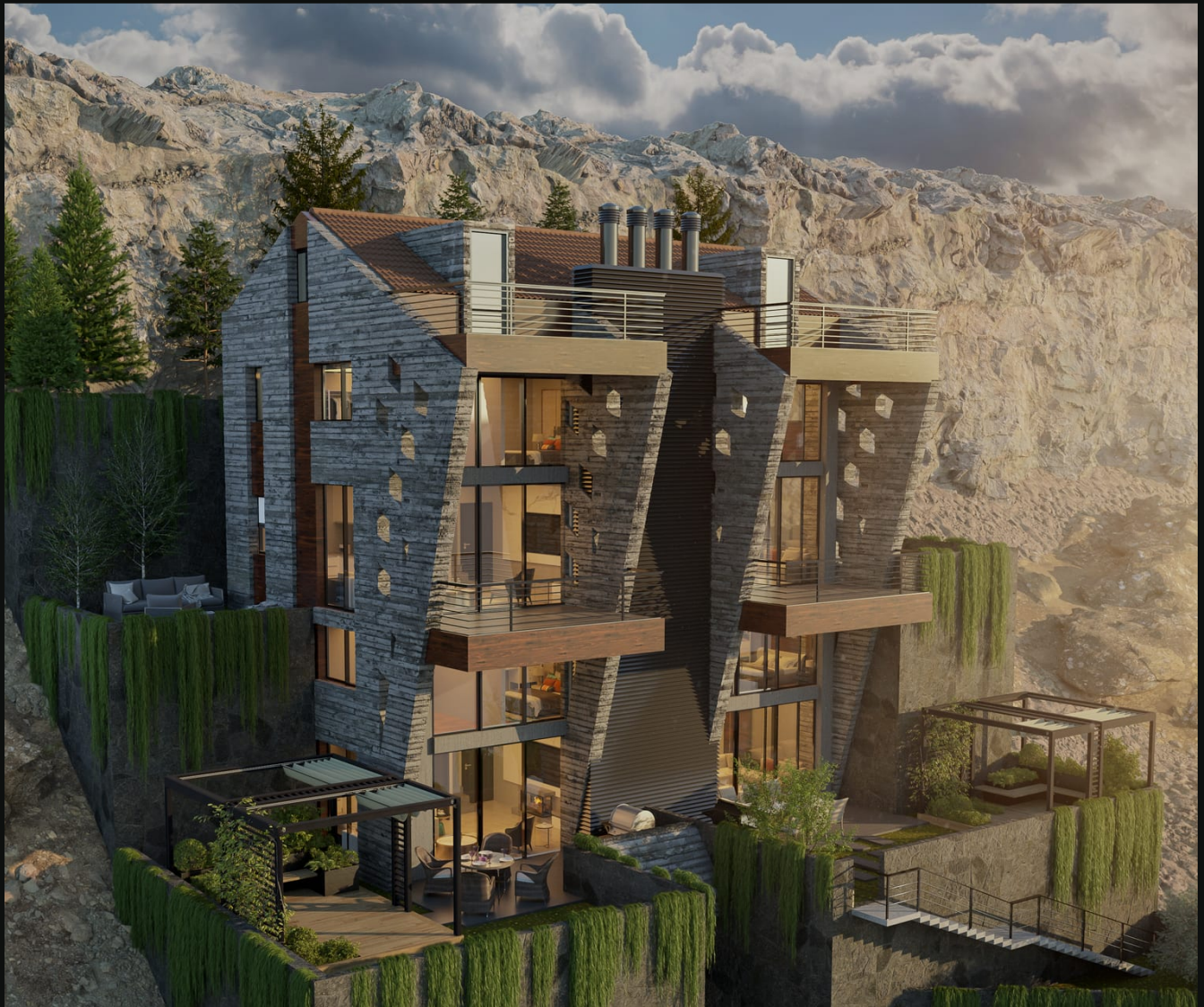
ASPEN 1 — BATTERED STONE PIERS STEPPING DOWN THE ROCK FACE
